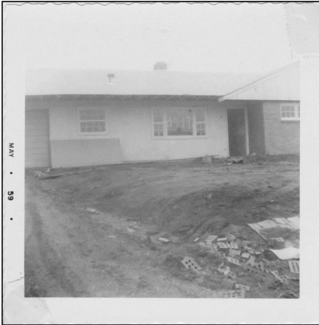
162 Cushwa Drive under construction. Photo courtesy of the Bombeck family.
